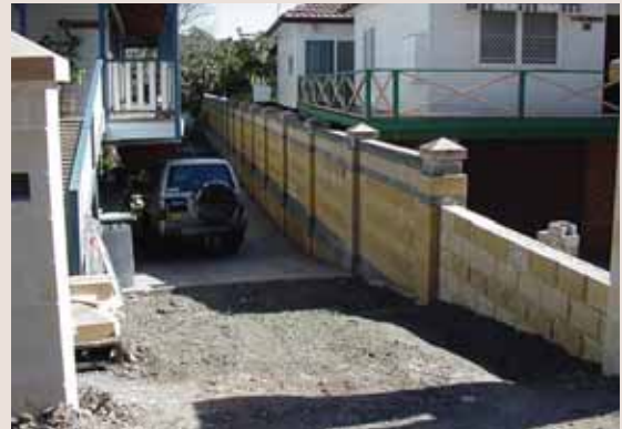
Figure 33 Boundary Fence and Velocity Reduction Barrier
