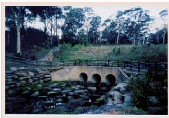
Figure 80 A typical outlet arrangement with natural rock velocity dissipators
