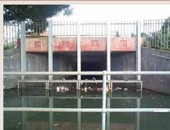
Figure 83 A typical Gross Pollutant Trap (GPT)
