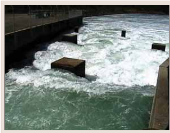
Figure 42 Velocity Dissipator in outlet channel
