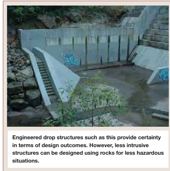
Figure 79 Drop Structure
