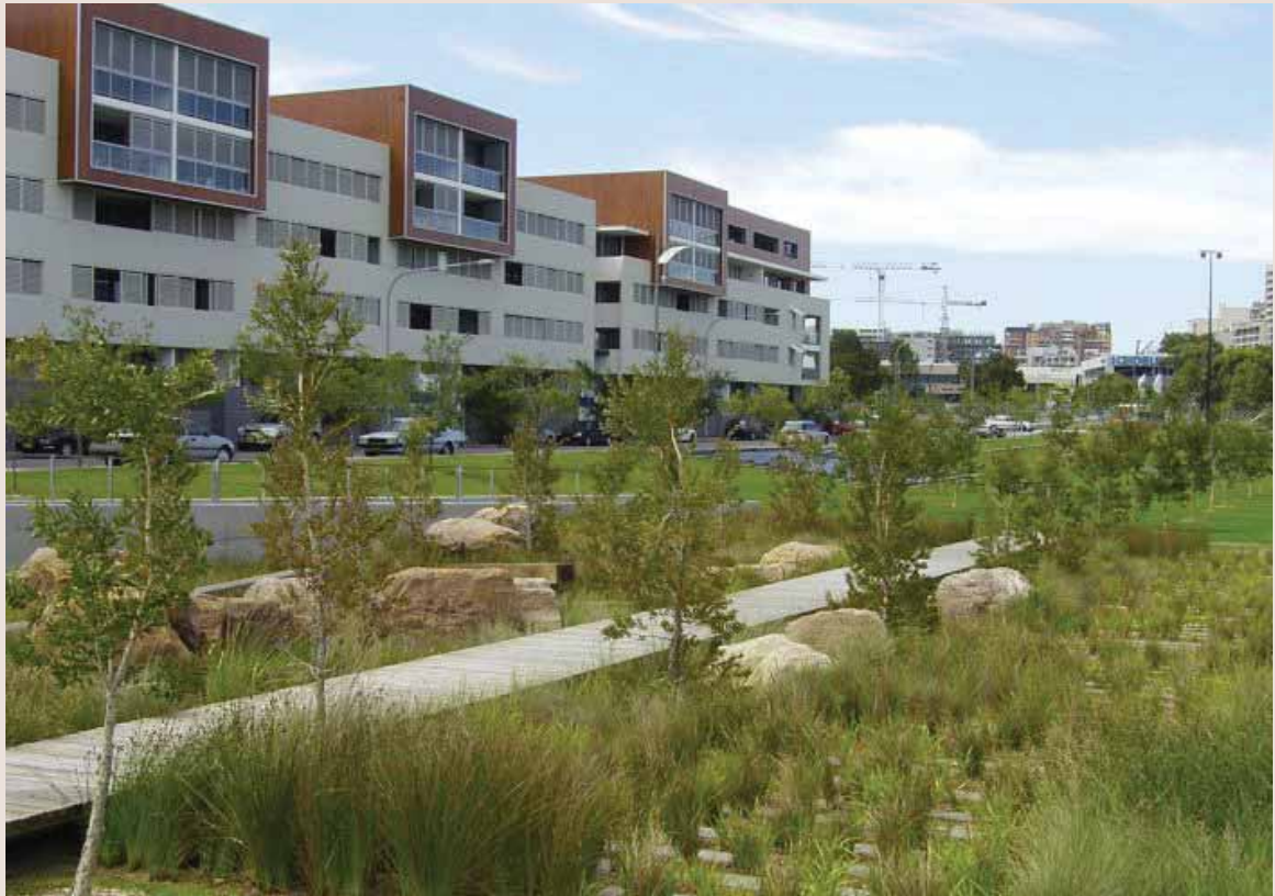
Figure 44 Integration of filtration system into a drainage corridor
