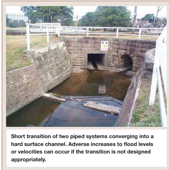
Figure 78 Channel – Pipes Transition
