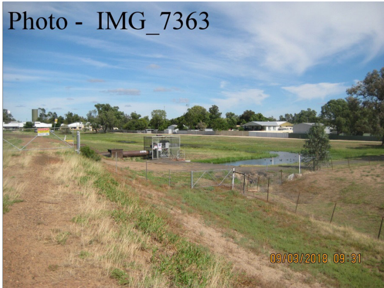
Ch. 3400 – Ponding Water at Town Side Toe
