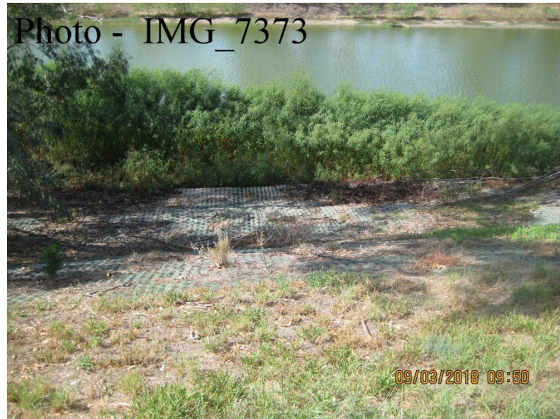
Ch. 4050 – Reno Mattress at River Side Toe
