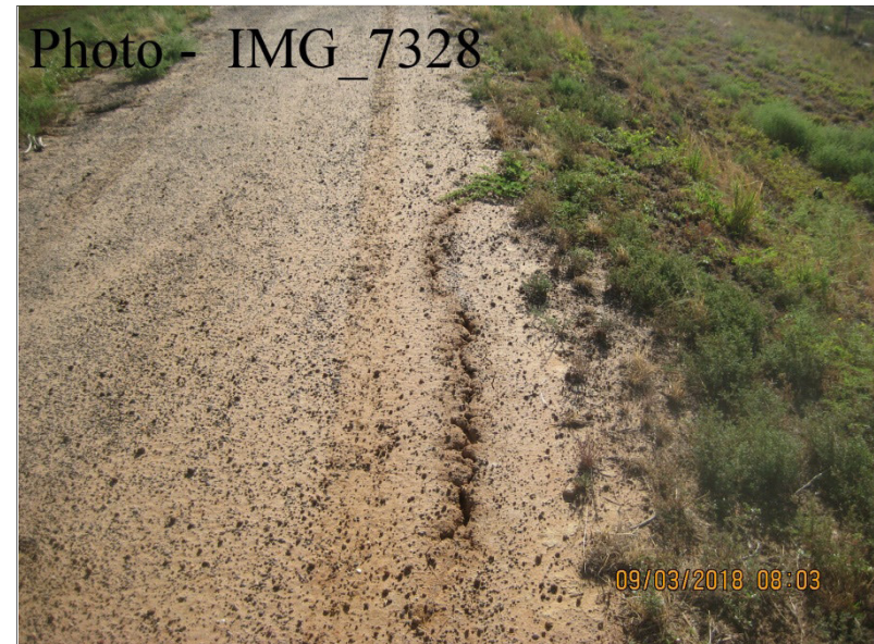
Ch 50.– Crack Town Side of Crest
