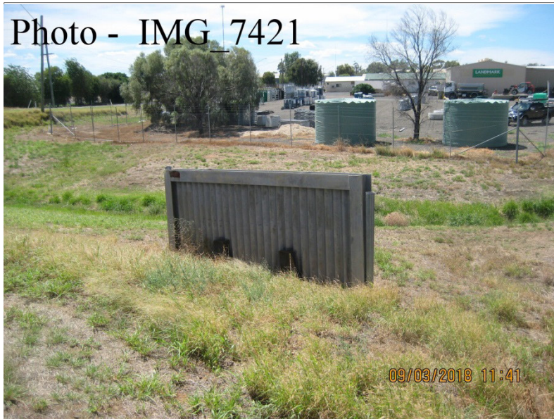
Ch. 6700 – Flood Gate for Western Rail Crossing
