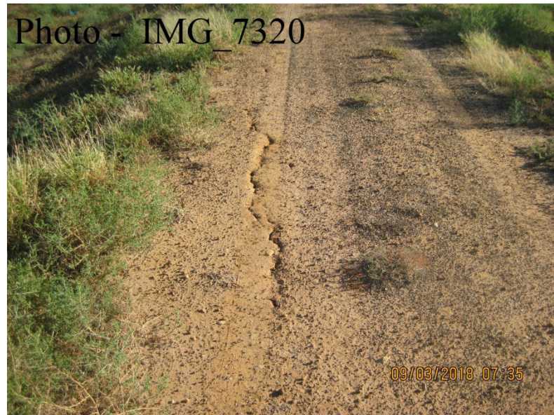
Ch. 7950 – Crack River Side of Crest
