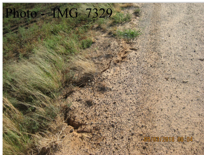
Ch. 50 – Crack River Side of Crest
