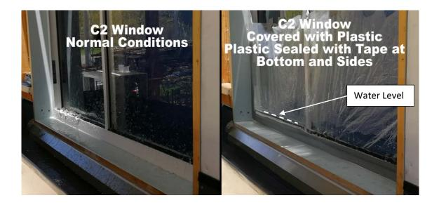
Despite this set-up some water can still leak through the tape or from above the window, you can place a towel on the window sill to absorb this water **<u>before</u>** the cyclone.
